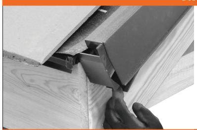
Place the **Natural Dry Verge Unit** on the tile and slide them down onto the **Eaves Stop End** ensuring that the fin has engaged.
